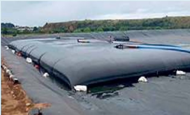
New Plymouth Wastewater Treatment Plant – Geobags
