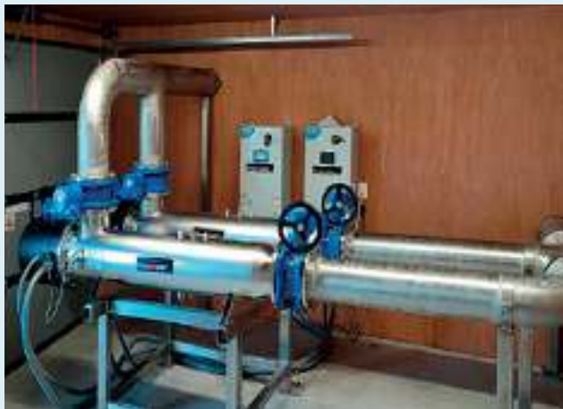
Kaikoura - Ultraviolet light reactors
