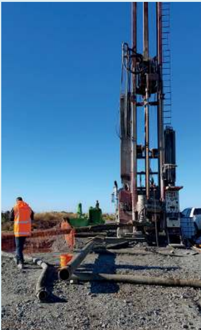
Invercargill – Production bore rig
