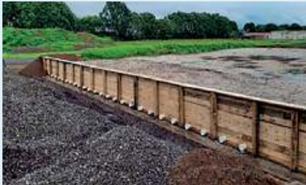
New Plymouth Wastewater Treatment Plant – Biofilter
