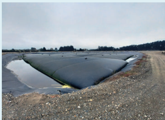
Hurunui District Council – Amberley wastewater ponds desludging to seepage bags
