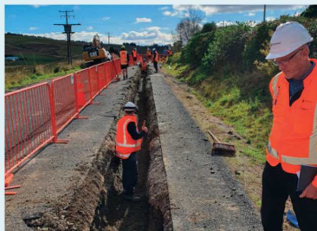
Dunedin City Council – Replacing the old lead jointed pipes in Waikouaiti Township.
