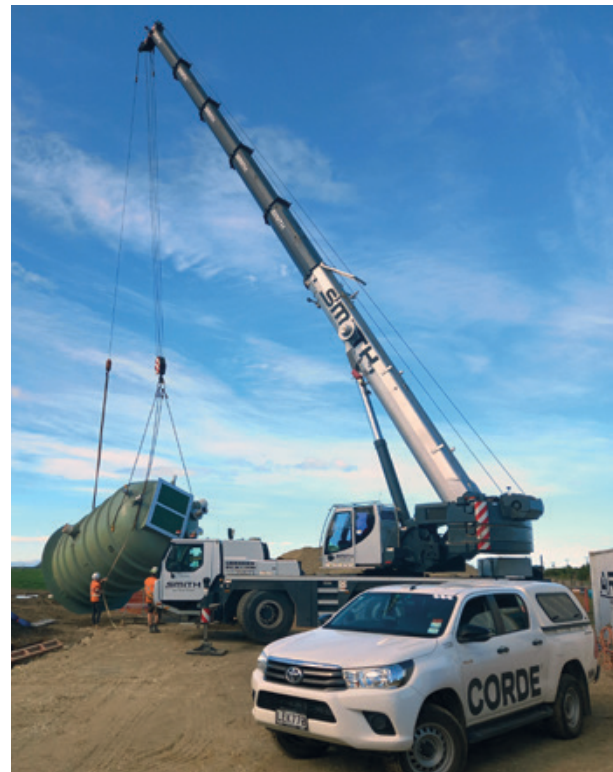
New pumpstation wetwell at Darfield - an important part of the overall scheme
