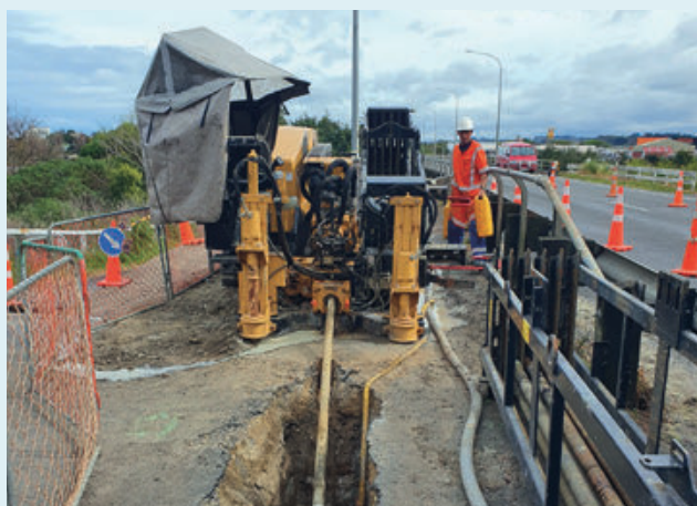
Whanganui District Council - Directional drilling, Cobham bridge (Airport Side)
