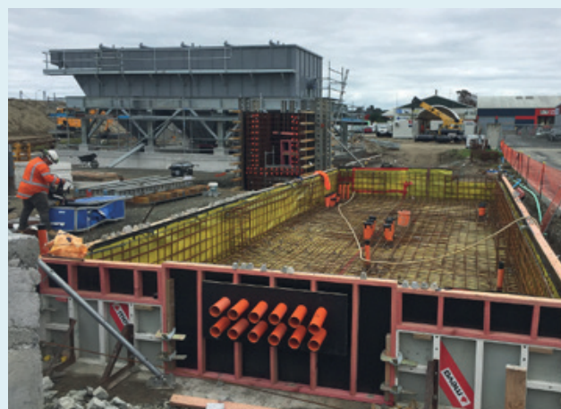
Gisborne City Council – Wastewater Treatment Plant clarifier and electrical building formwork
