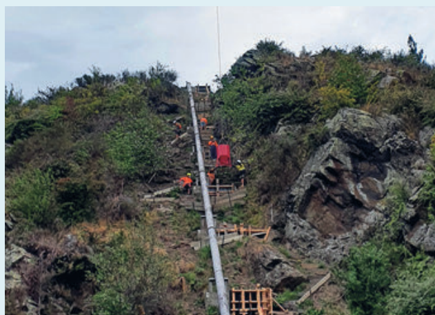
Central Otago District Council – Clyde Falling main water pipe replacements
