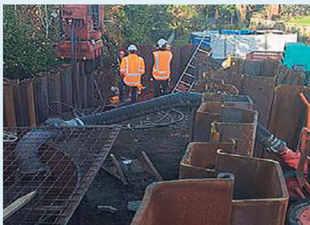
New Plymouth District Council - Waiwaka culvert sheet piling
