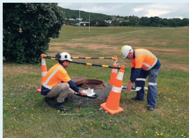
Porirua City Council – Very High Criticality Asset, pipe inspection in Titahi Bay
