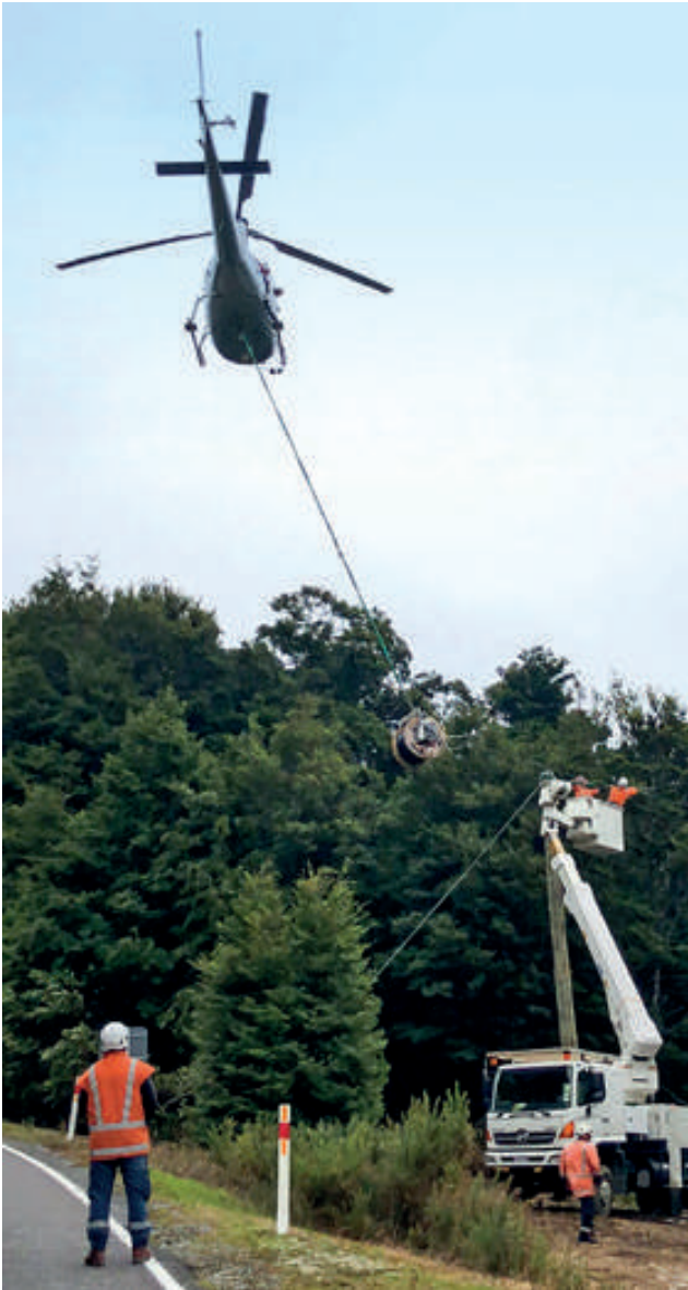
Helicopter laying fibre on an aerial section of the route
