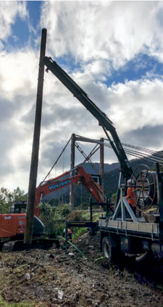
Erecting a pole for an aerial fibre river crossing, Jacobs River
