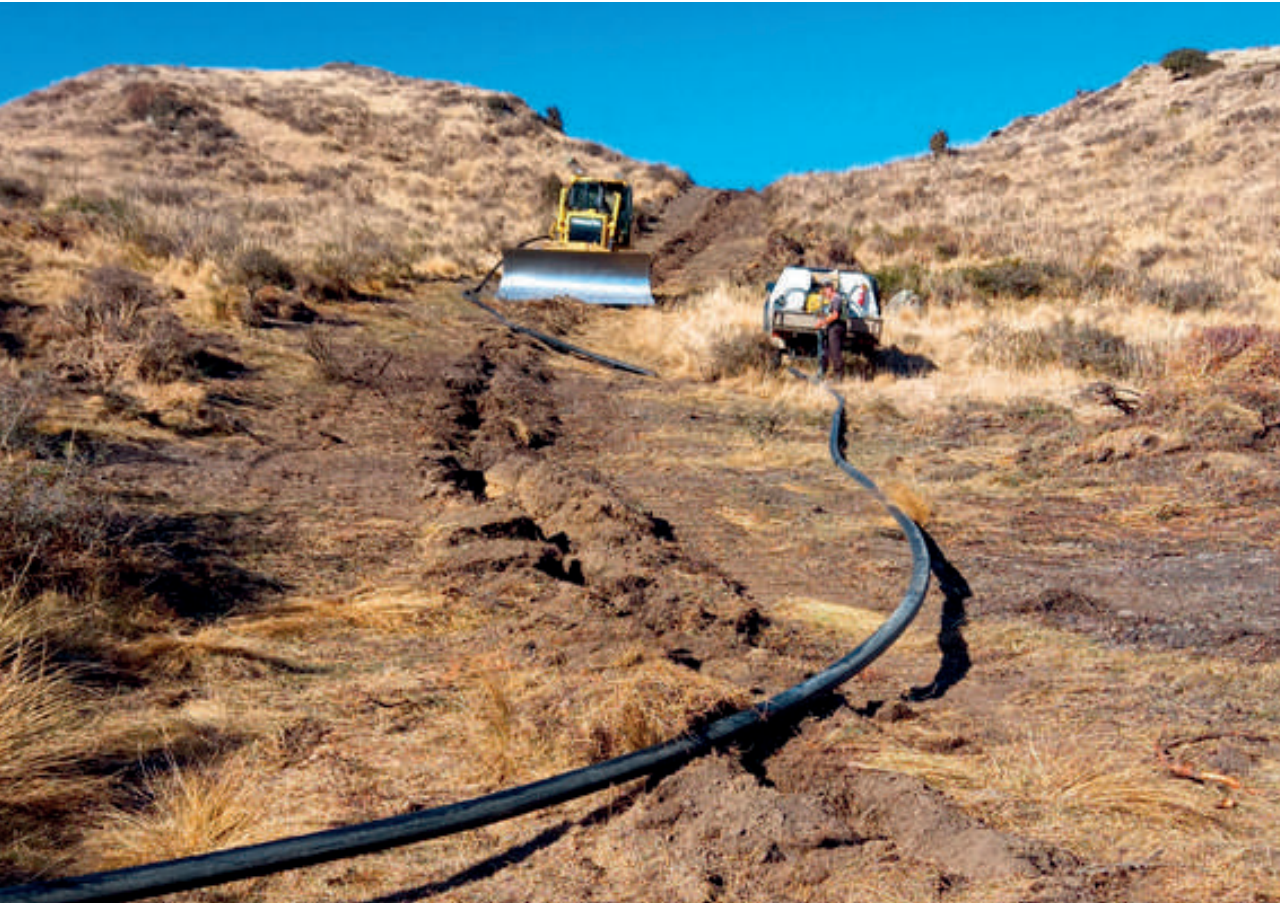
Pipe Laying using mole plough technique on Mt Alexander, Glendhu in the Hurunui District
