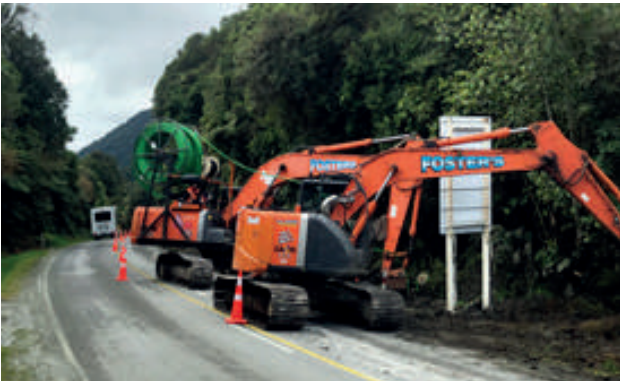
Diggers at work laying underground duct for the fibre on Haast Highway
