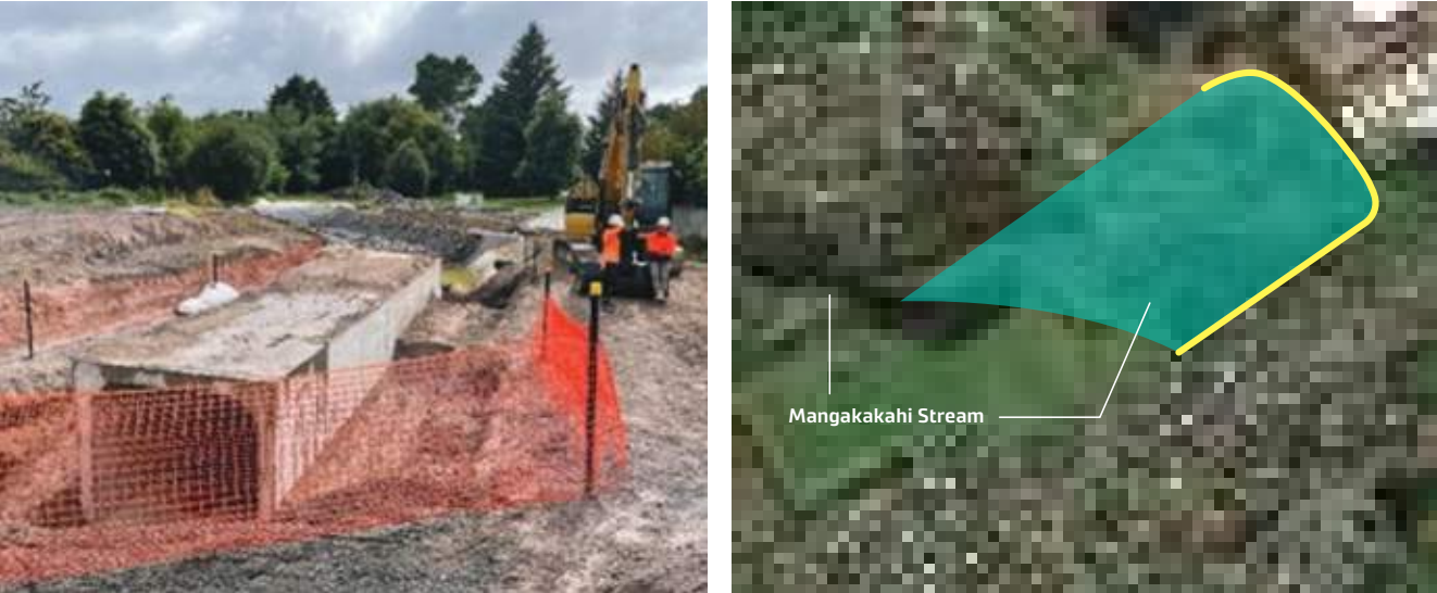
Linton Park detention dam in construction. The new dam provides increased flood mitigation and allow for future development within the community.
