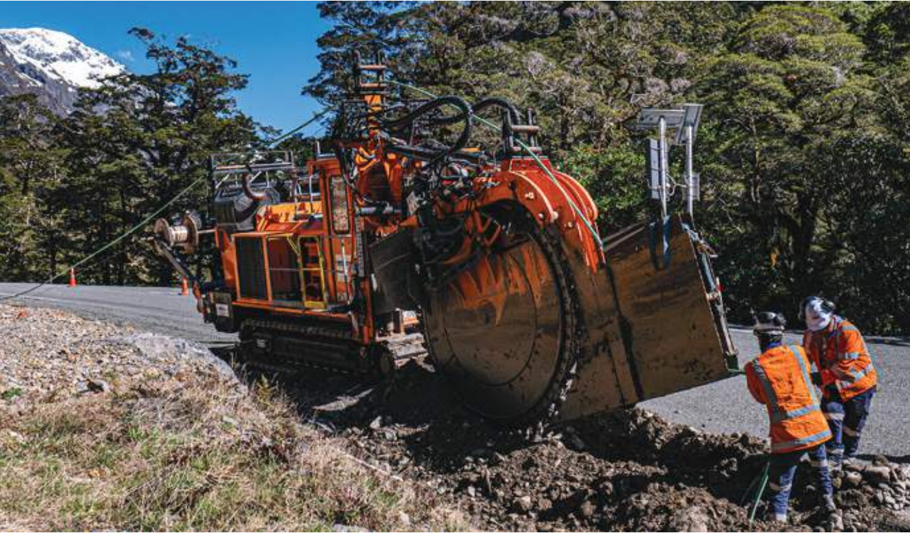
Rock Saw busy laying fibre along SH94 to Milford
