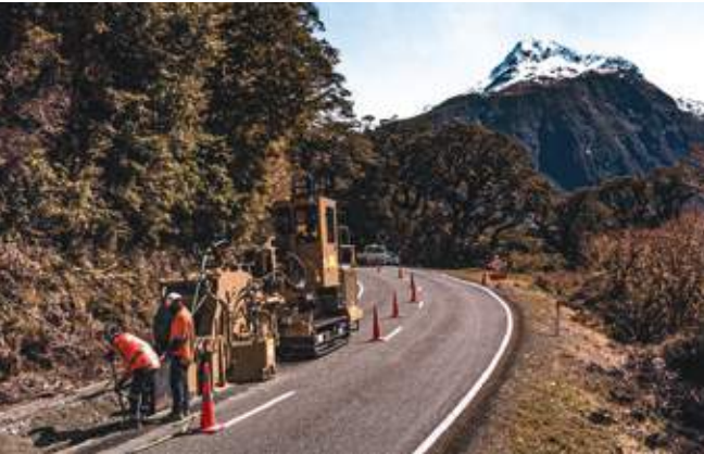
Crew laying fibre on SH94
