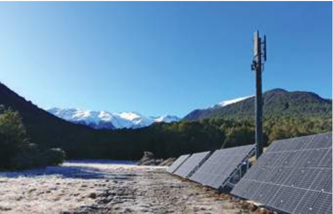
Tower at Mirror Lake, SH94, showing the solar panels for the off-grid power supply
