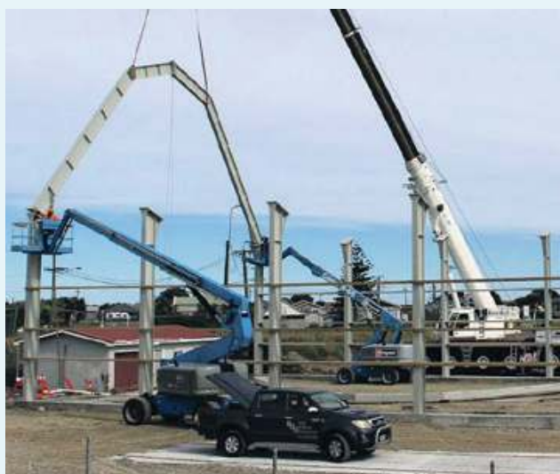
Greymouth Slipway Shed first roof support installation
