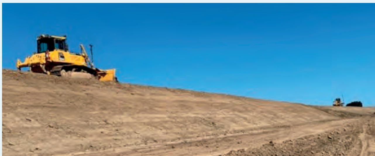
Waipaoa River Flood Control - dirt transfer on to the top of the stop bank
