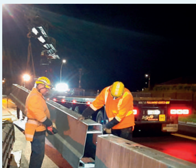
Rotorua SH30 Upgrade, Night works Safety barriers
