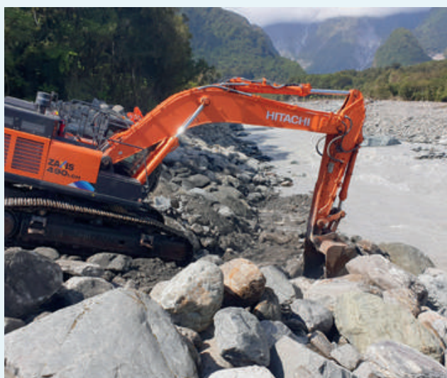
Fox River Reinstatement – Rock Armour being undertaken to protect the exposed landfill site
