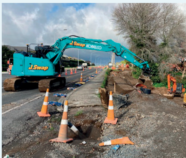
Omokoroa, fill over power duct
