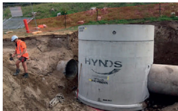
Installation of the Defender Unit as part of the Hawai Street Stormwater project.
