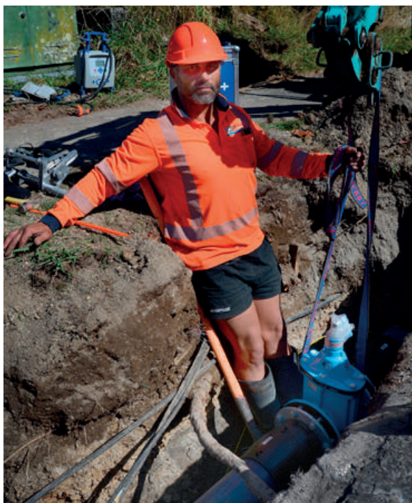
Valve installation for water network renewals.
