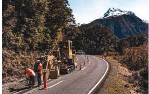
Crew laying fibre on SH94
